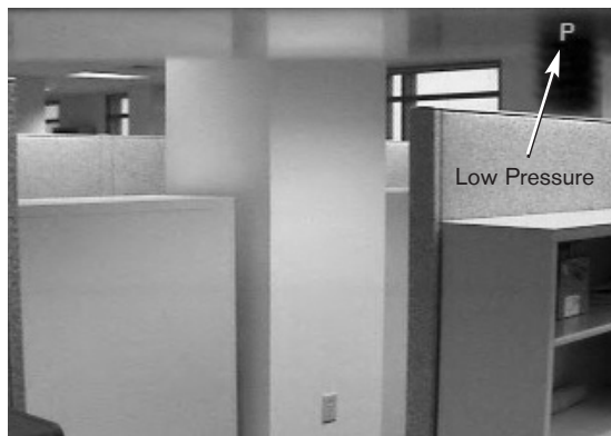
Photo 7D Low Pressure Alarm continued
